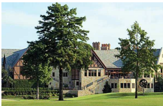
Clubhouse on the Polish Country Club course – contemporary view.
